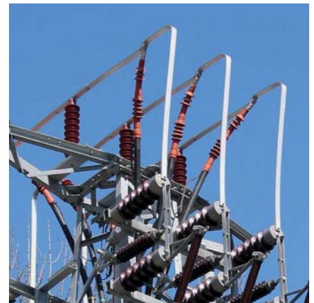
Raychem TFT 42 kV outdoor terminations
