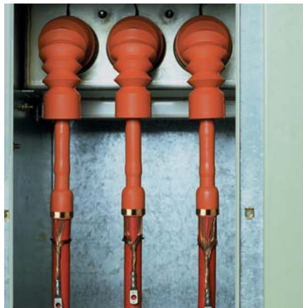
Raychem TFTI terminations installed with Raychem bushing boot (RCAB)
